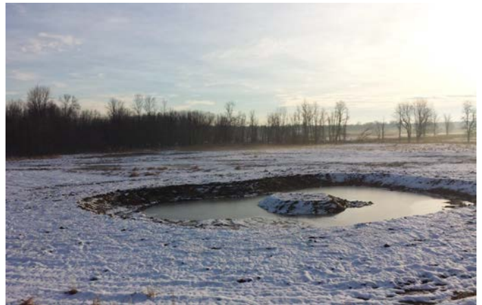
Below: the new ponds at this location after construction.
